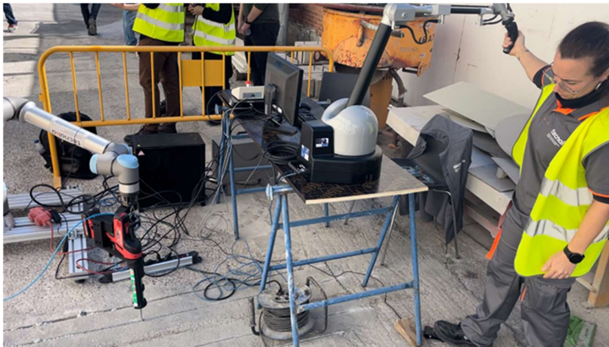
Figure 16 Image for the robotic setup on site during the integration workshop
