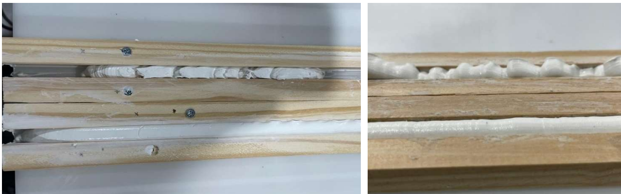
Figure 15 Real joint filling. Teleoperated demonstration above, automatic filling below for joint 2.
