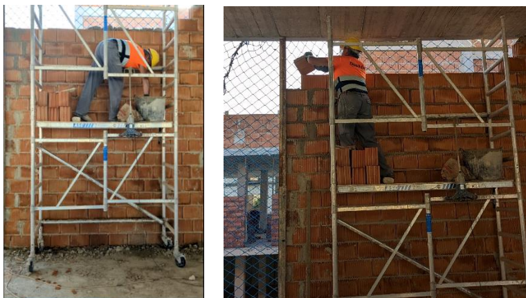
Figure 6 – A bricklayer at two different moments of its routine. Bricklaying is highly repetitive task which risk injury increases with weight and when working below knee (on the left) and above shoulder (on the right).
